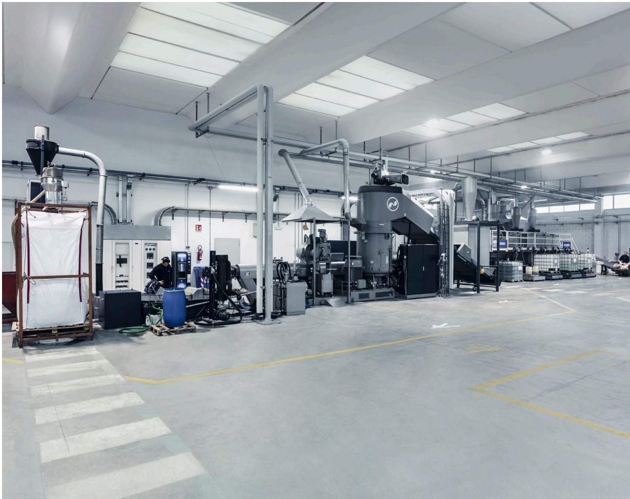
Front view of the Santa Margherita production line.
